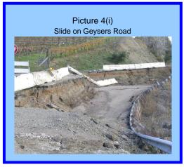
repaired, to prevent future washouts. Damaged roadway features, including pavement and base/sub-base, guardrail, and signs or markers, are repaired or replaced. The area may also be re-vegetated or buttressed with rock or walls to protect steep natural slopes.
